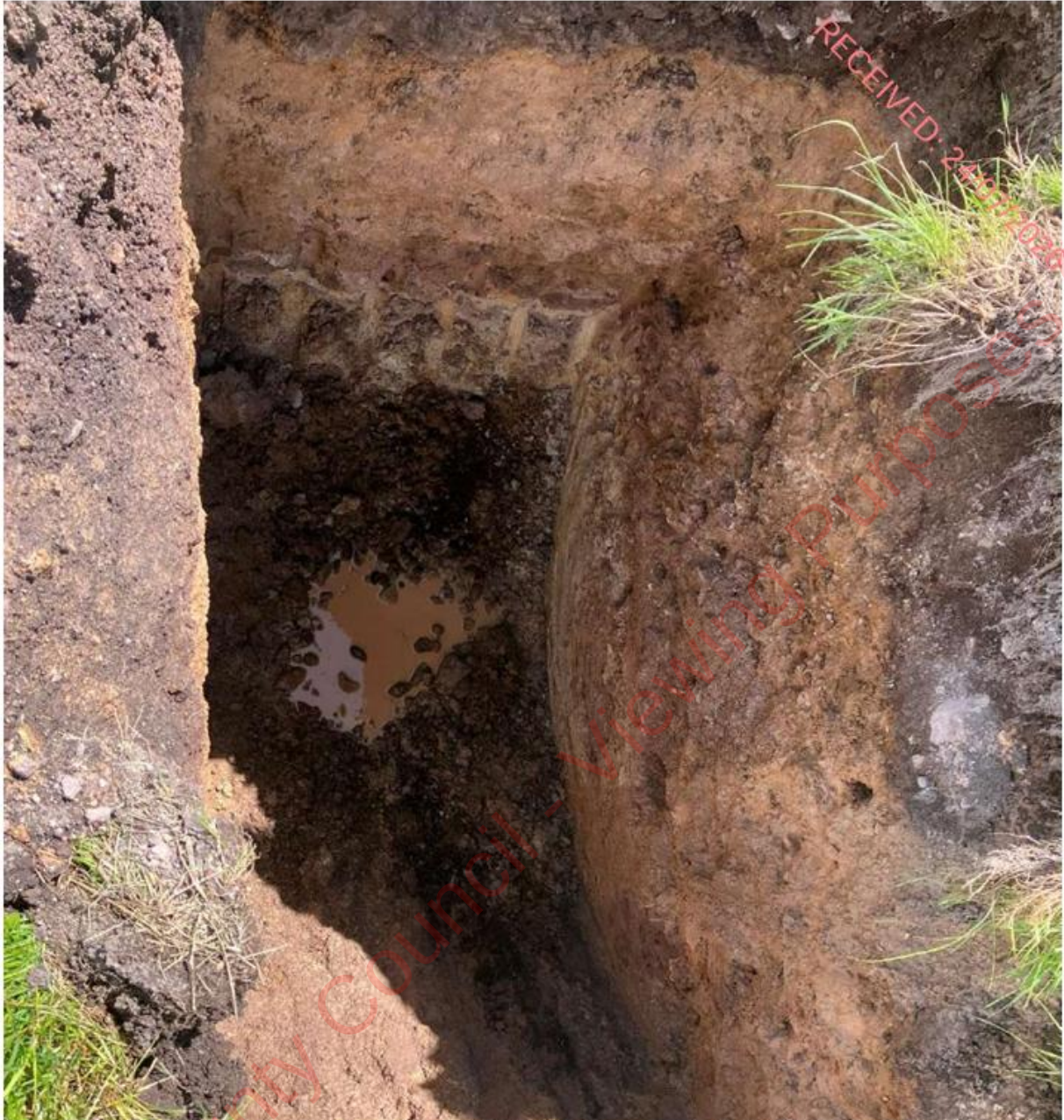
Fig: Trial Hole as dug
