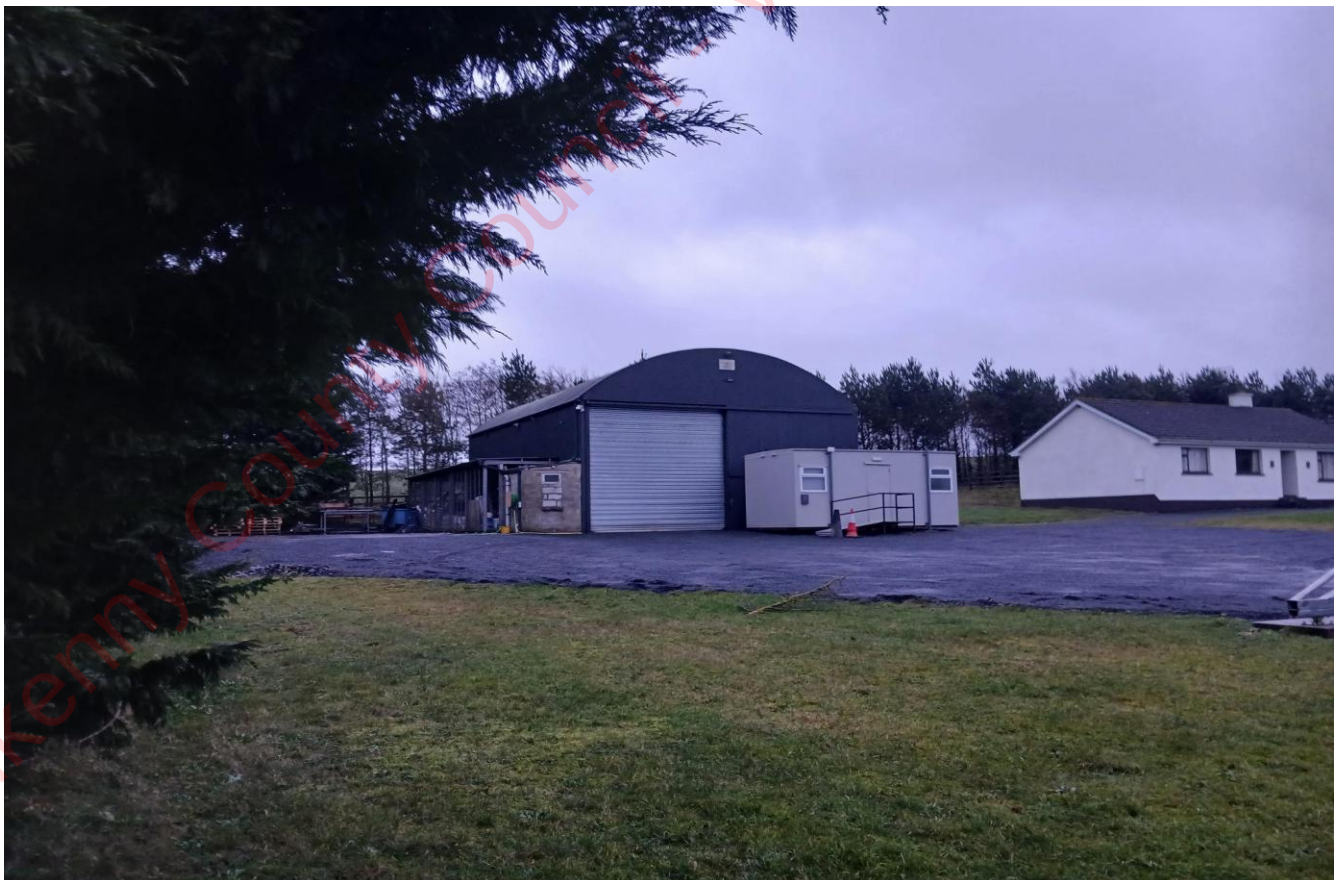
Planning Inspection Photos dated 14 th January 2026
