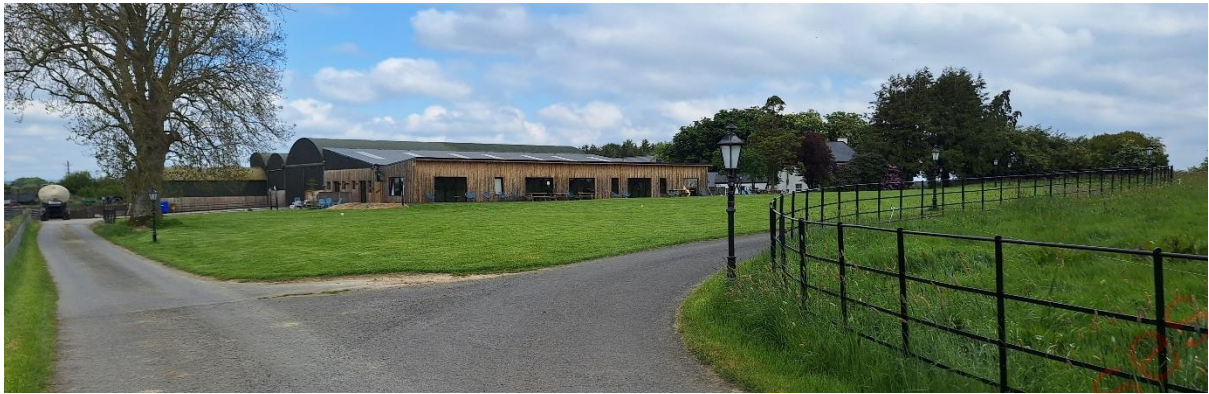
Photo of activity centre, units 5 and 6, and farm buildings from the driveway
