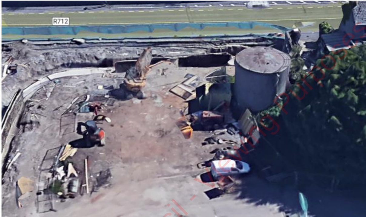
Legacy tank -likely left over from the former Cattle Mart
