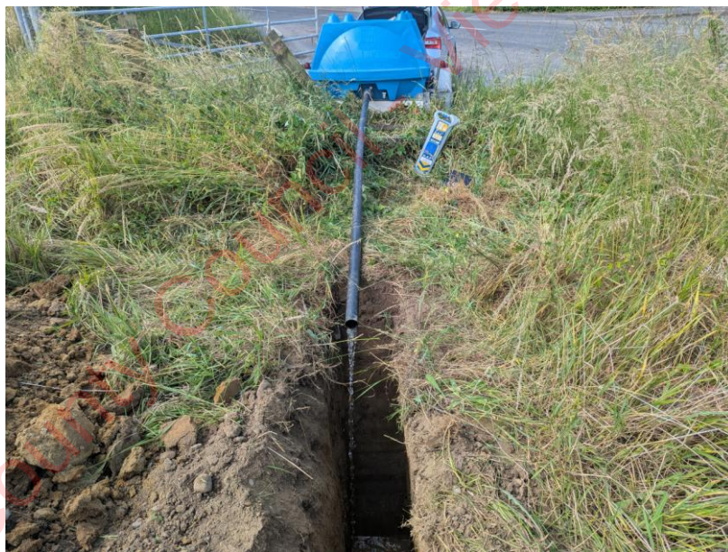
Figure 4. Filling ST1 with water
