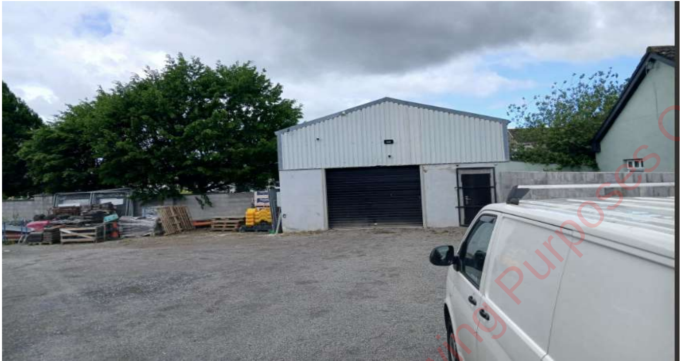
Planning Inspection photos dated 4 th June 2026.
